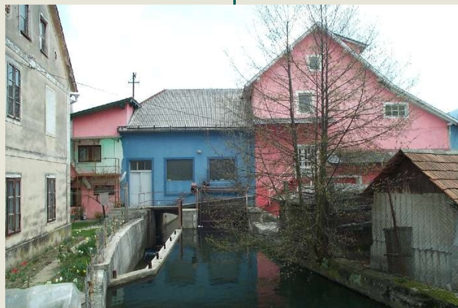
vodna elektrarna – nekdaj imenovana Vrbenka hydroelectric power plant – formerly known as Vrbenka
